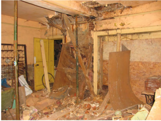
2013 Northwold Manor. Central block, inner hall, view south-east.
