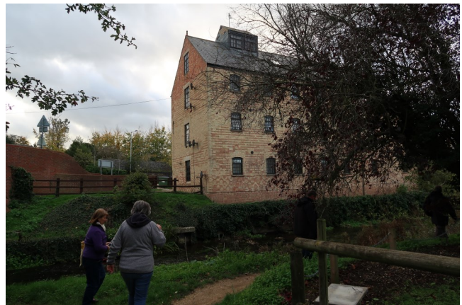
The old mill now converted for modern residential use.
