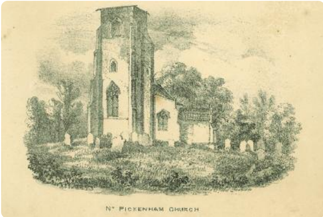
St. Andrew's Church, North Pickenham, was rebuilt in 1863.
