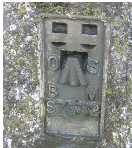
Plate on side, showing OSBM and ref no. for trigpoint at Shingham Heath
