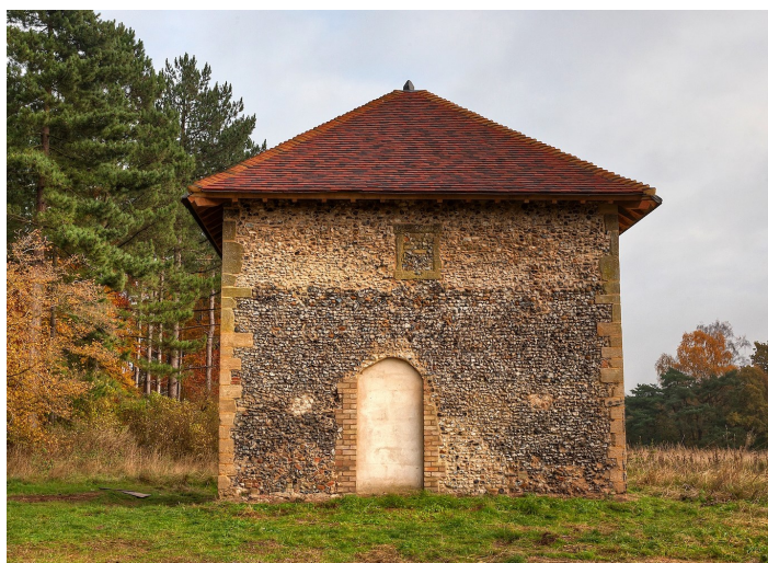
Mildenhall Warren Lodge, with its new roof
