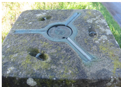
Top of trig pillar at Drymere, showing mounting for a theodolite and lines of sight to other trig stations
